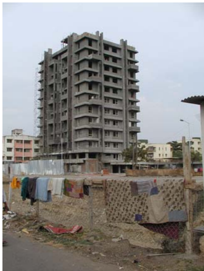
Baustelle Sylvan Heights in Aundh/Pune
